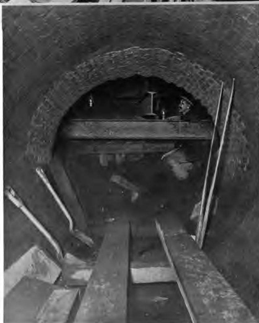
SPECIAL CONSTRUCTION OF 6 1/2-FOOT SEWER, UNDER CHATHAM SQUARE
